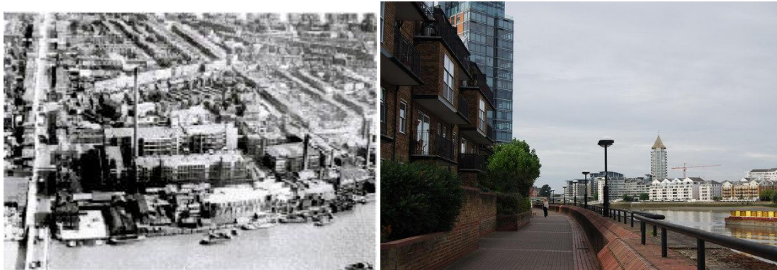
Fig. 2: (L) Morgan Crucible epitomised Battersea's riverside industries in the 1950s, viewed in aerial shot from above Chelsea. (R) The Thames Path in Battersea today, next to housing redevelopment on the same site, walking westward from Battersea Bridge and looking across the river to the postmodernist tower on the Chelsea Harbour estate.
